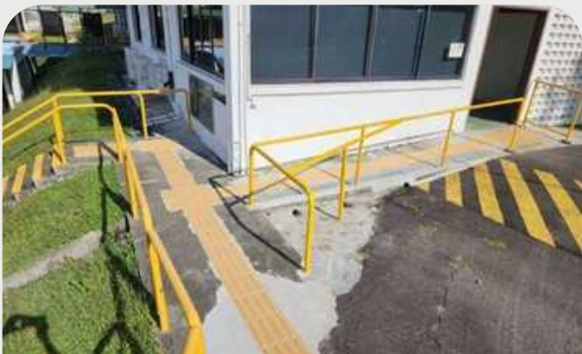
New tactile tiles & handrails realignment at DCC Building
